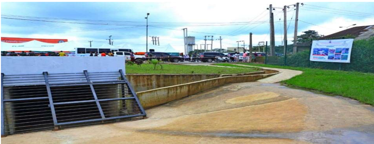
Figure 4: Functional concrete-lined gutter on Shelter Afrique/IBB corridor, exemplifying how modern drainage enables clear roads and smoother transportation
